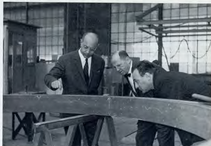
One of the steel stiffening rings used to reinforce the PX-15 pressure hull gets a critical look from David Bannerman, center, of the American Bureau of Shipping, at the Monthey construction site. The PX-15 is the first submersible to be certified by ABS.
