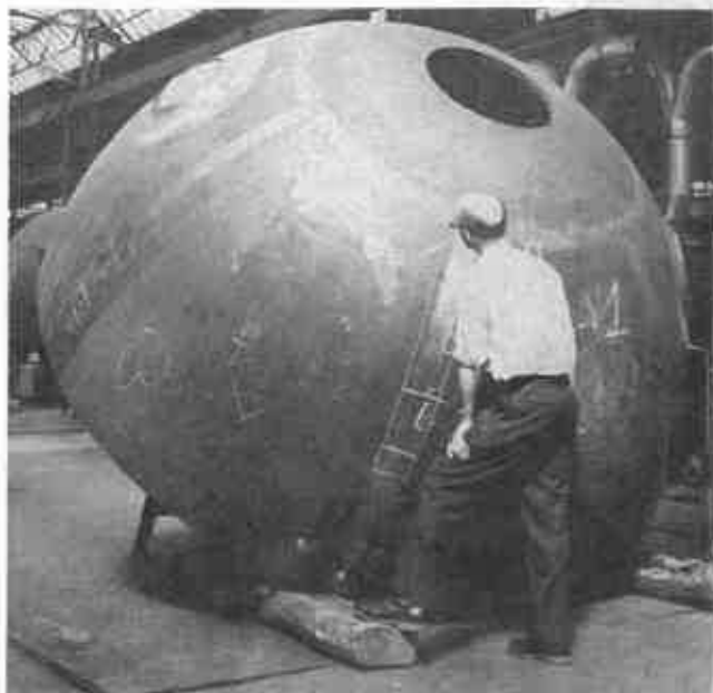
Fig. 5—Technician checks completed hemispherical section. Chalk marks identify X-ray film locations.
